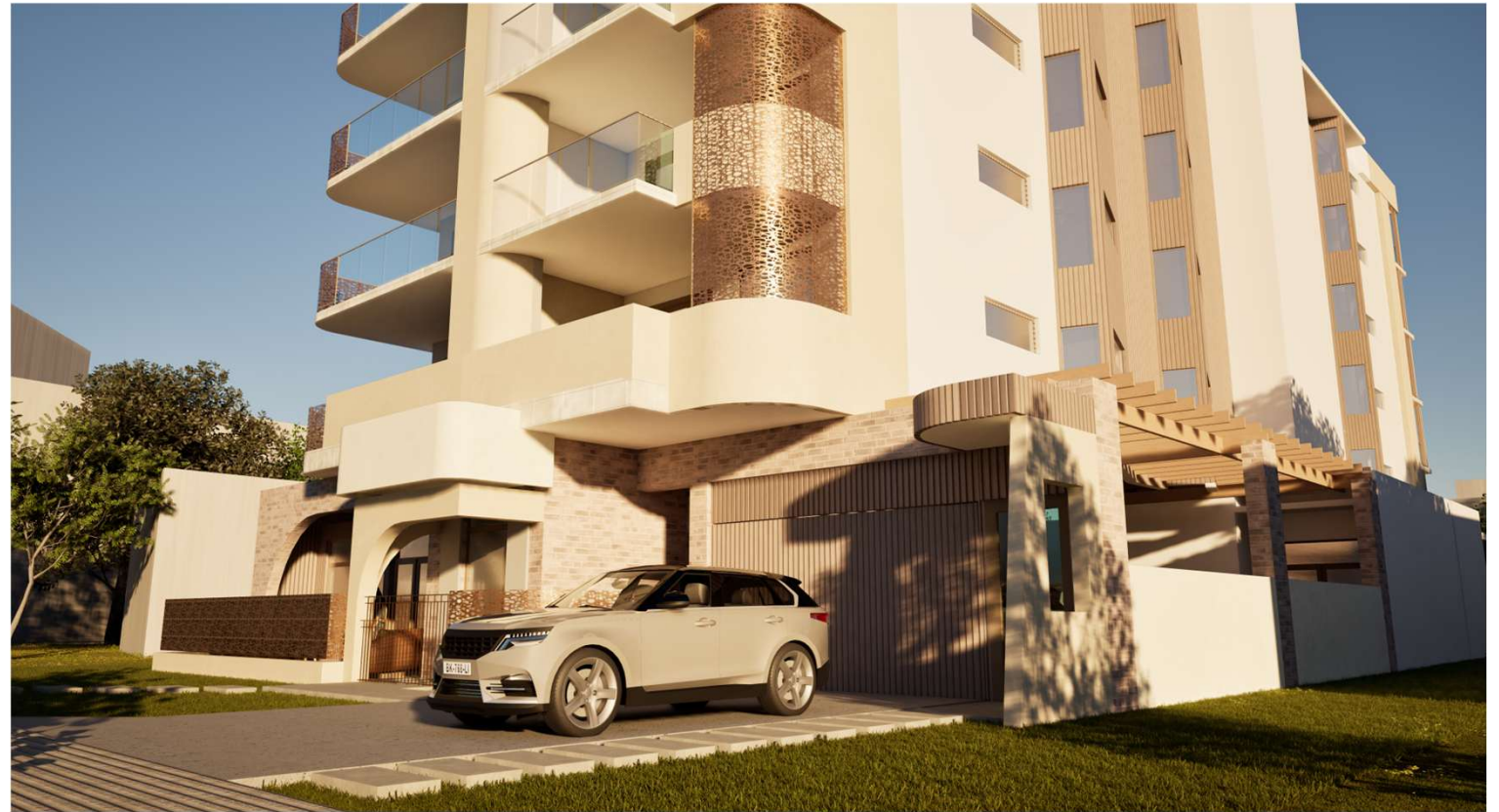
Entry to Building
