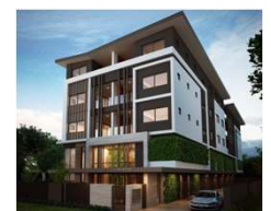
Apartment block 21 Kishorn Street
