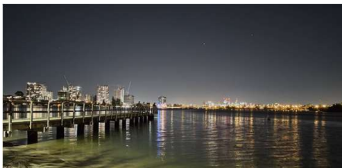
Deep Water Point Jetty
